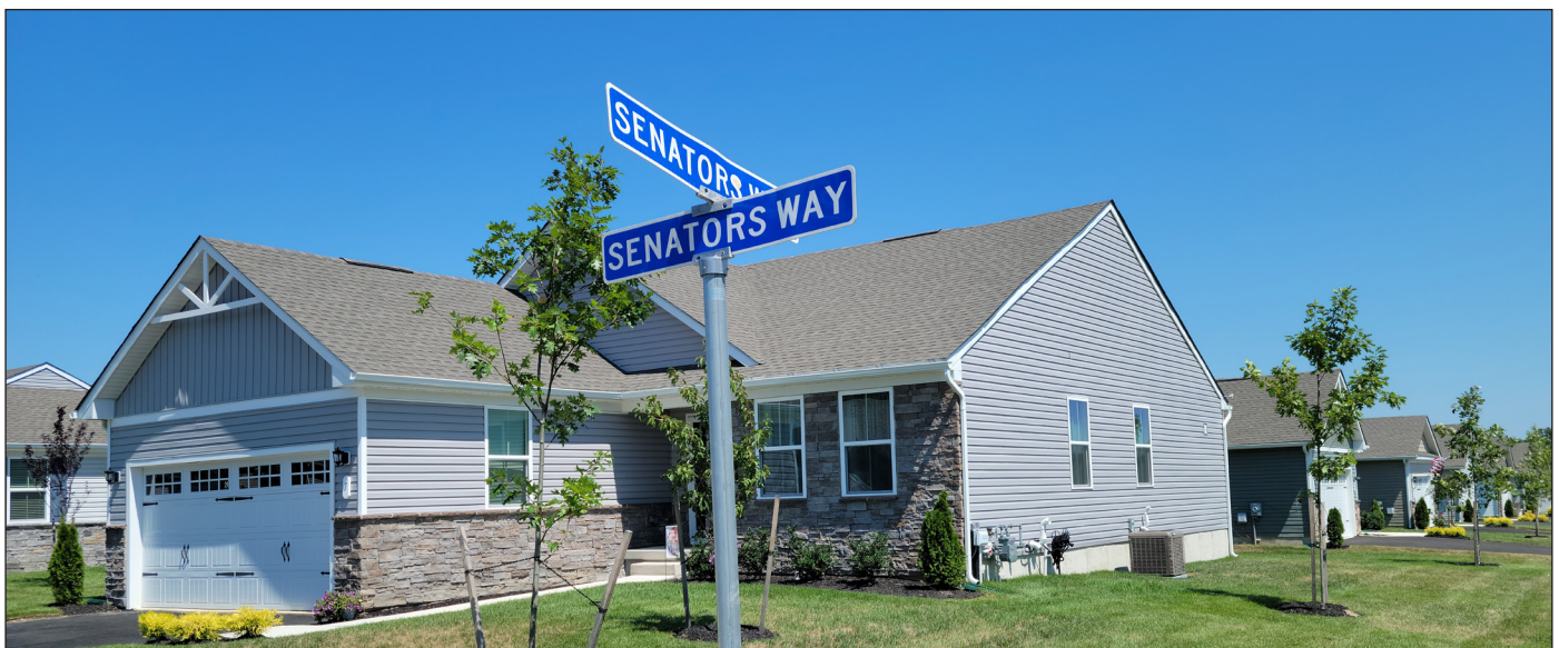
Above: This 94-unit, single-family housing development in Winslow Township, Camden County, was built with the use of 6 Pinelands Development Credits (PDCs), including 3.25 PDCs that were redeemed in February 2022. Photo/Paul Leakan
