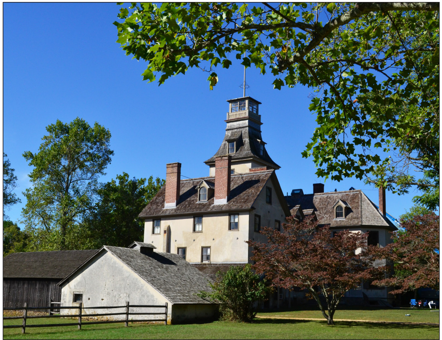
Above: The Pinelands Commission approved 32 applications for public development in 2022, including the installation of a geothermal well field for the heating and cooling of the historic Batsto Mansion.
